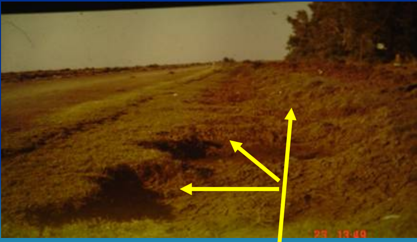
Inadequate Sedimentation Clearance
