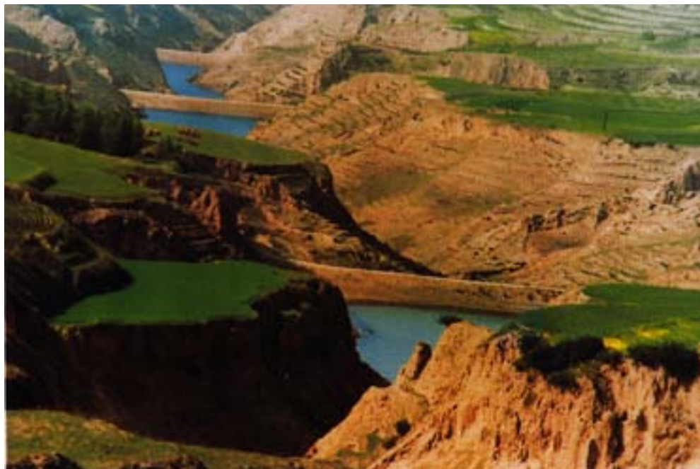
Figure 3 Key Dams for Gully Erosion Control
