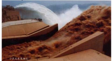
Fig. 7 Flood Released from the Xiaolangdi Reservoir for Regulation of Water and Sediment Downstream
